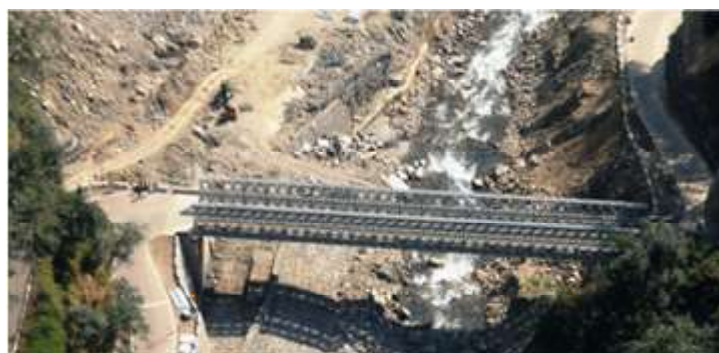
The 60m, double lane, permanent ACROW bridge launched in record time at Sonprayag, en-route to the Kedarnath Shrine. (Mar 2016)
